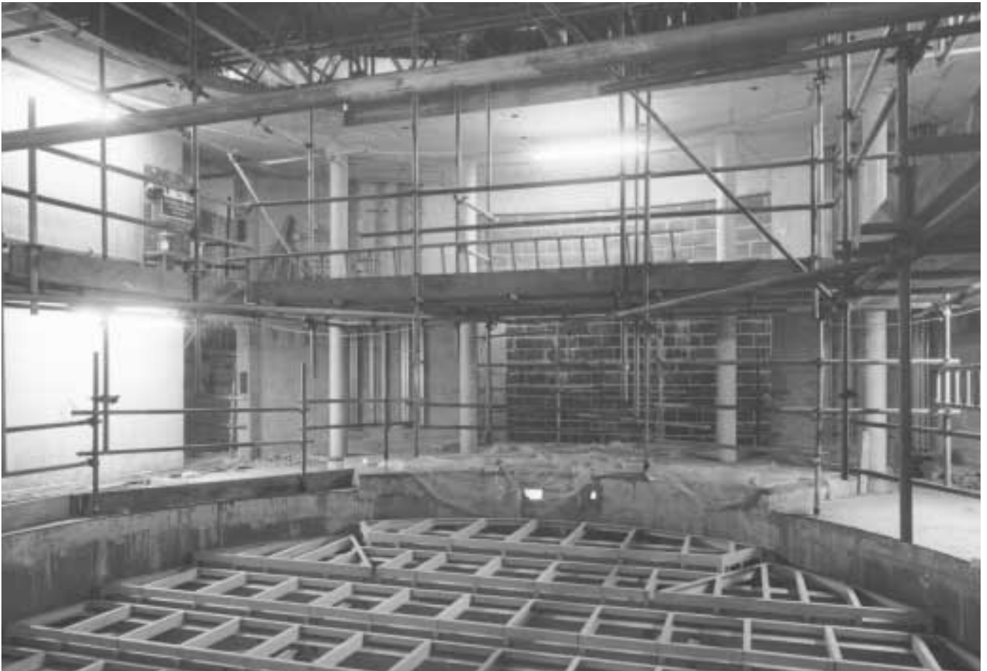
The new Vanbrugh auditorium – the actors view from the stage with moveable stalls floor structure in the foreground
