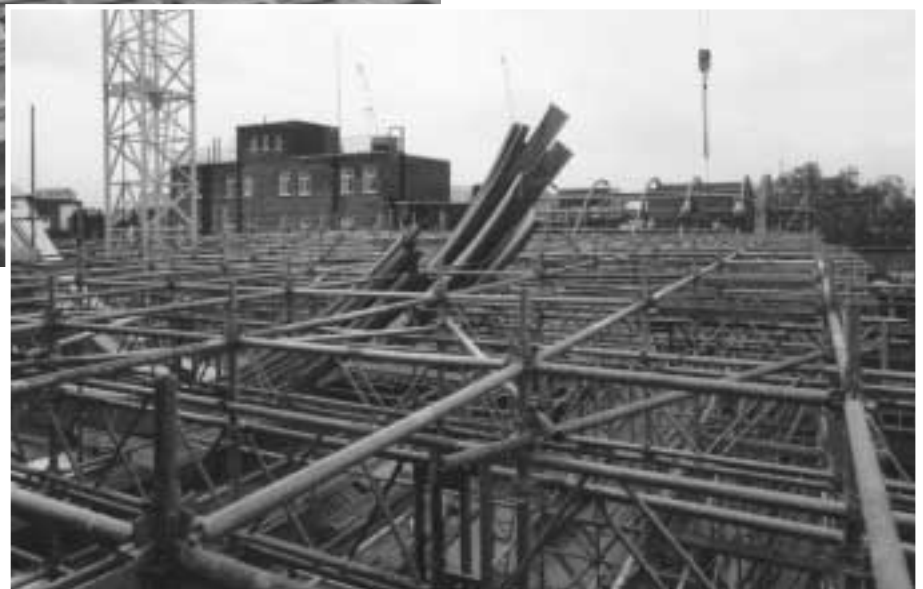
The vast temporary structure over the barrel vault roof
