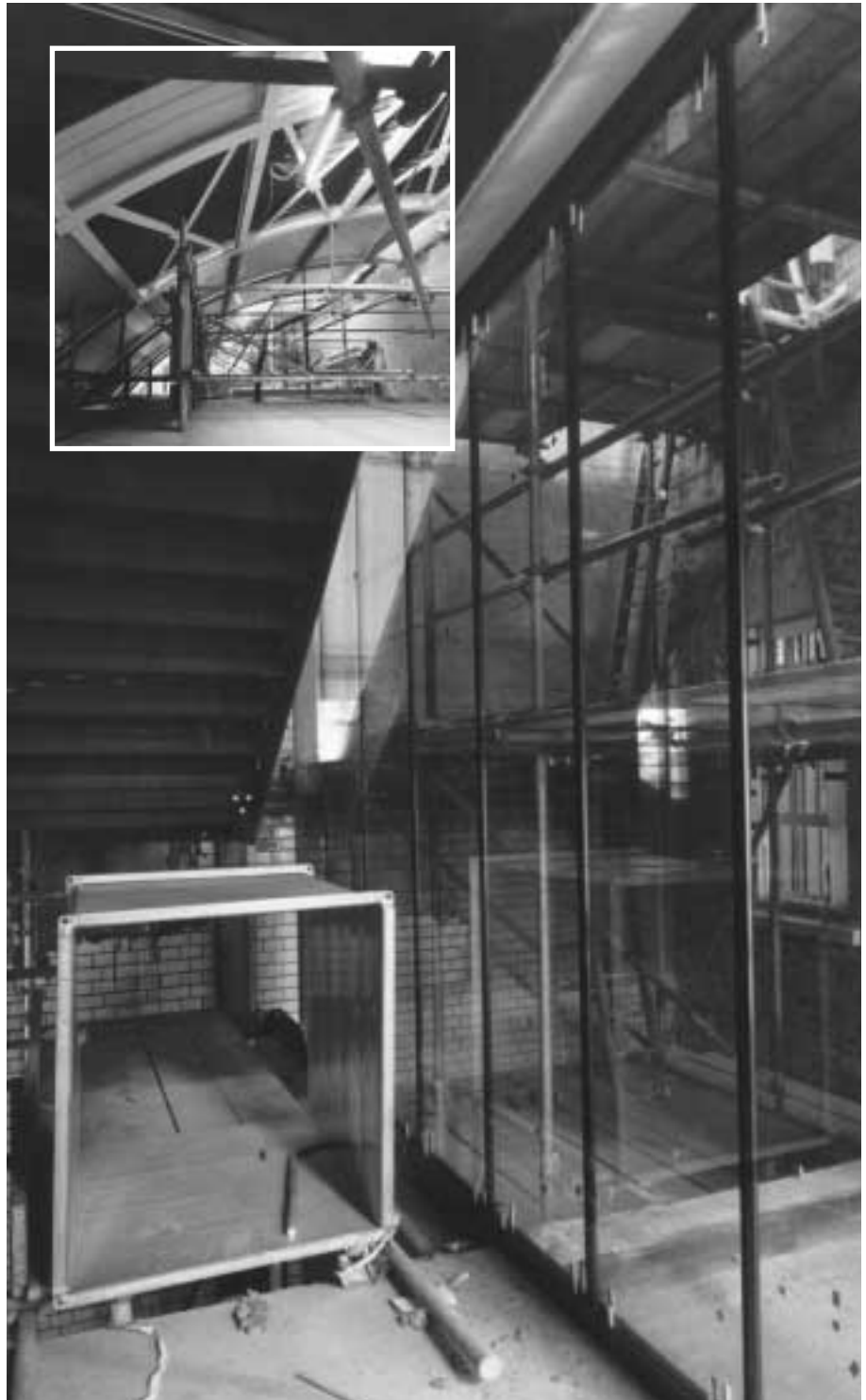
The glazed open lightwell – with inset showing the underside of barrel vault roof
